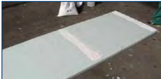
3. Apply two strips per panel (GIPSCOLL consumption: approx. 600 g per strip).
