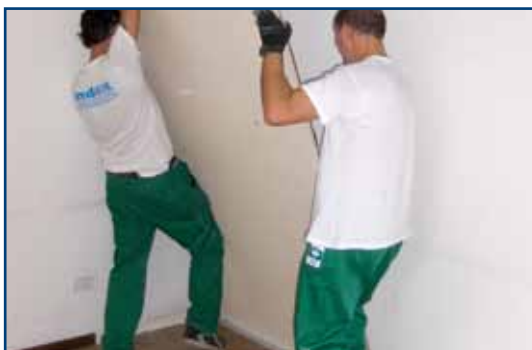
3. Put the panel of TOPSILENTDuogips in position
