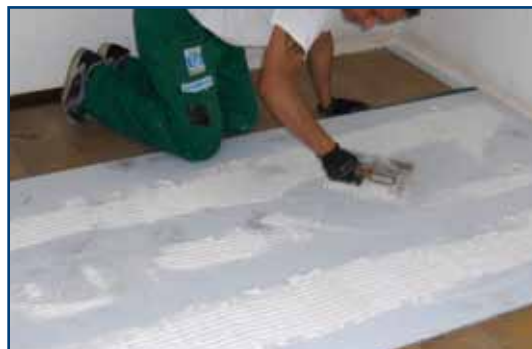
2. Spread the GIPSCOLL glue on the panel
