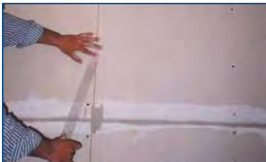
5. Lay and seal of plasterboard
