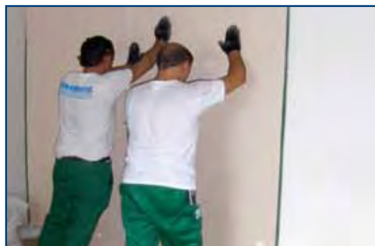
4. Put another panel of TOPSILENTDuogips in position
