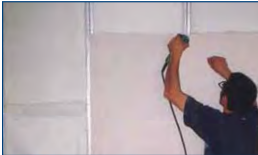
3. First layer of plasterboard
