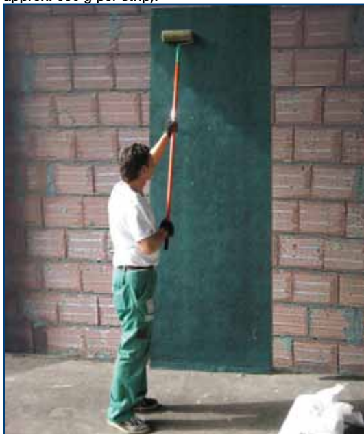
5. Press the panel using a painter's roller.
