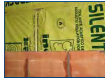
Erecting the 2 nd brick wall
