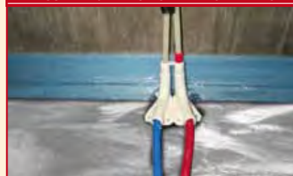
INSULATING DEVICE OF VERTICAL PIPES
