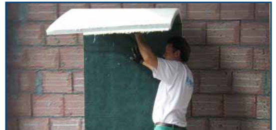
4. Place the panel on the wall.
