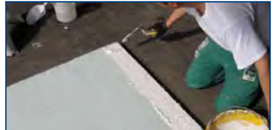
2. Spread with a spatula on the wool of TOPSILENTEco.
