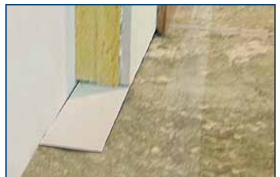
2. Position the sealing strip
