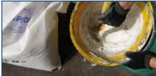
1. Mix the powder glue GIPSCOLL with water.
